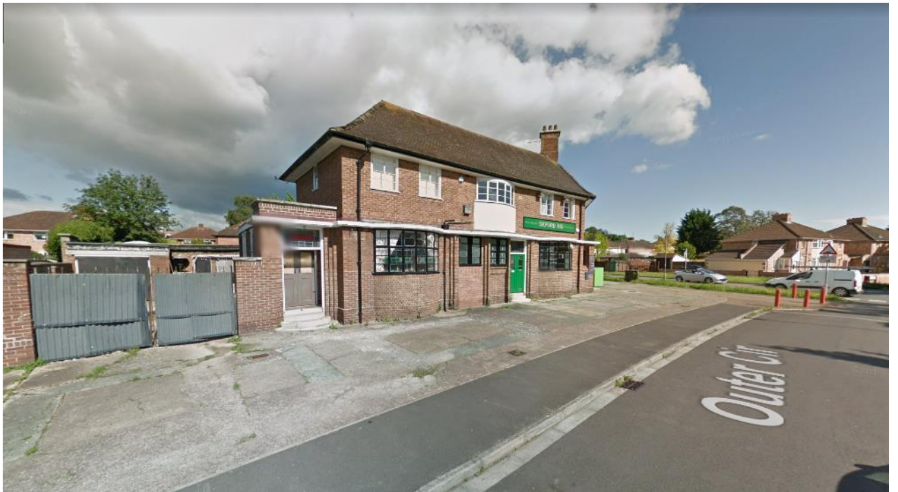
Looking East towards Roman Road
